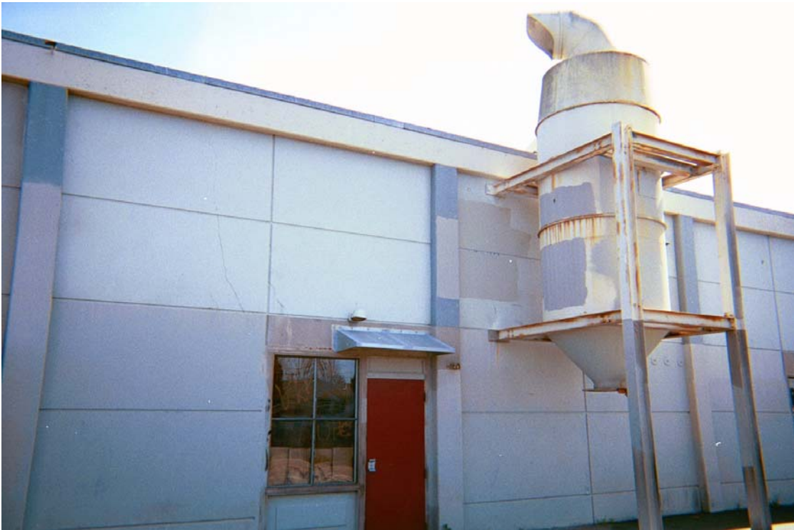
Figure 10: West Wall of Unit B
