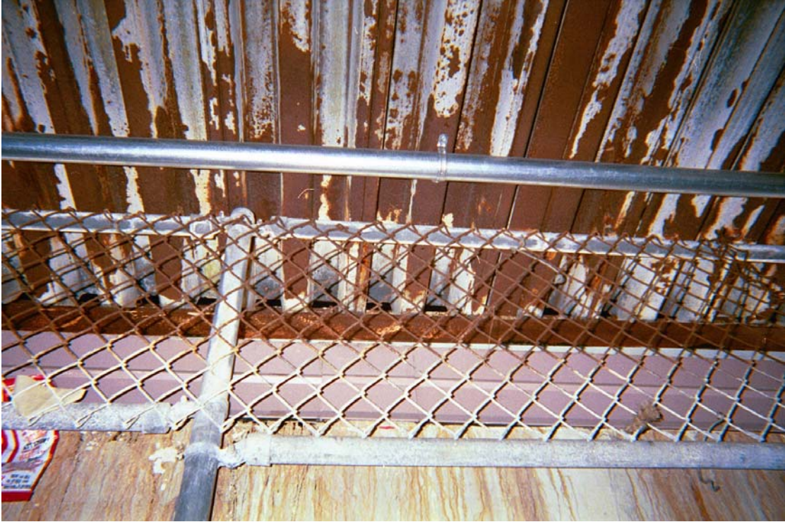
Figure 13: Metal roof adjacent to Cafeteria.
