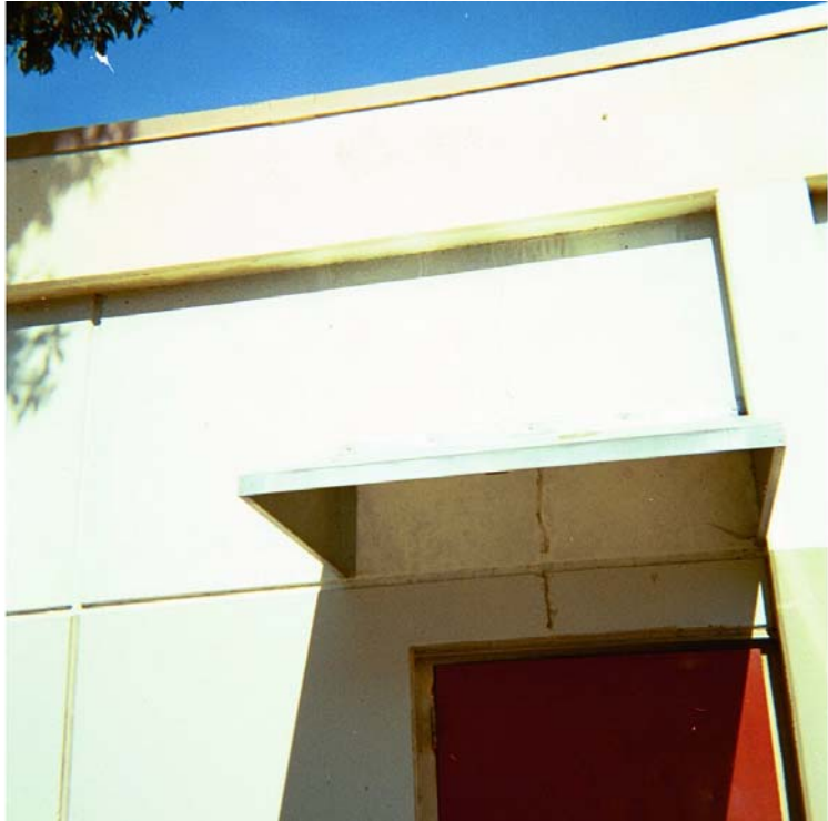
Figure 11: South Wall Unit D
