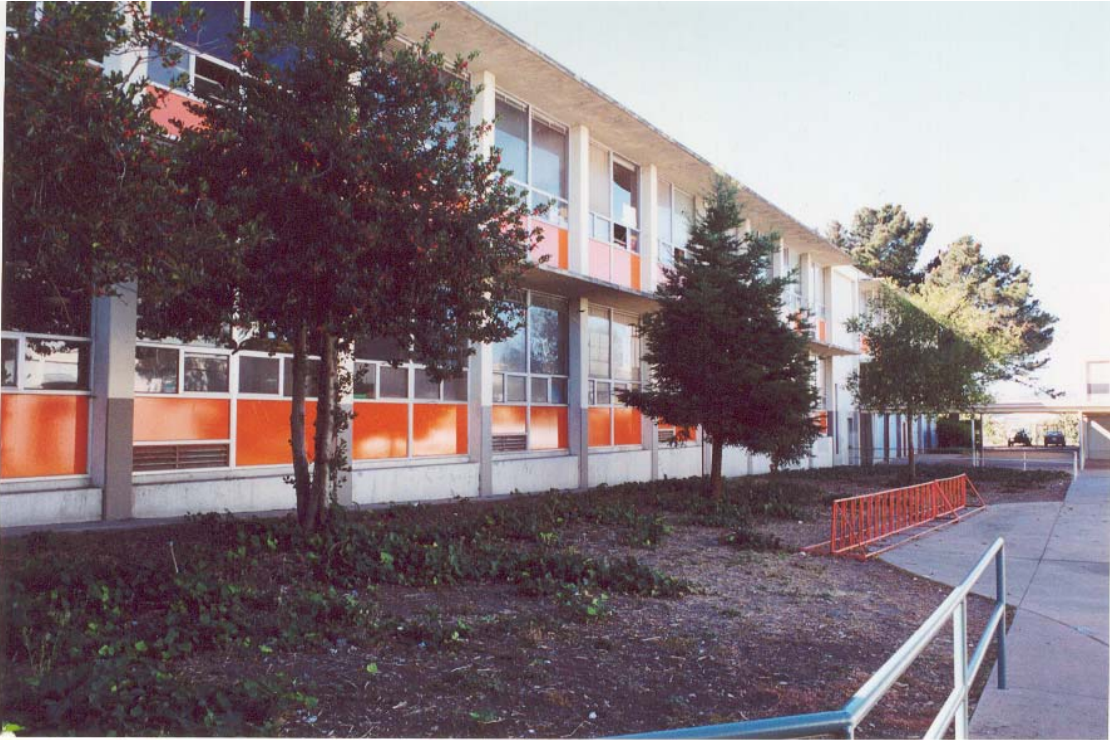
Figure 4: North Side of Classroom Building
